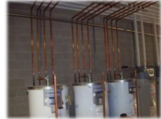
Heat Recovery - Refrigeration Units $0.28 per kWh annual savings
