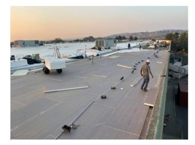
Roof Insulation is installed on top of the roof R30 Min
