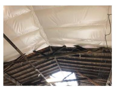
Attic Insulation is installed interior or under the roof R30 Min
