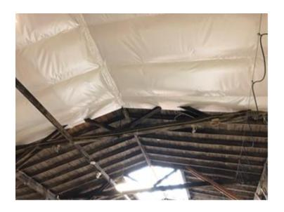
Attic insulation is installed in the interior or under the roof R30 Min
